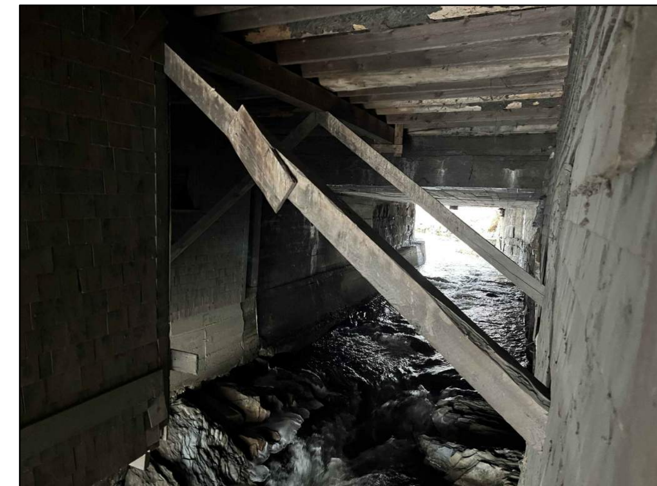
PHOTO 4 DOWNSTREAM LOOKING UPSTREAM
