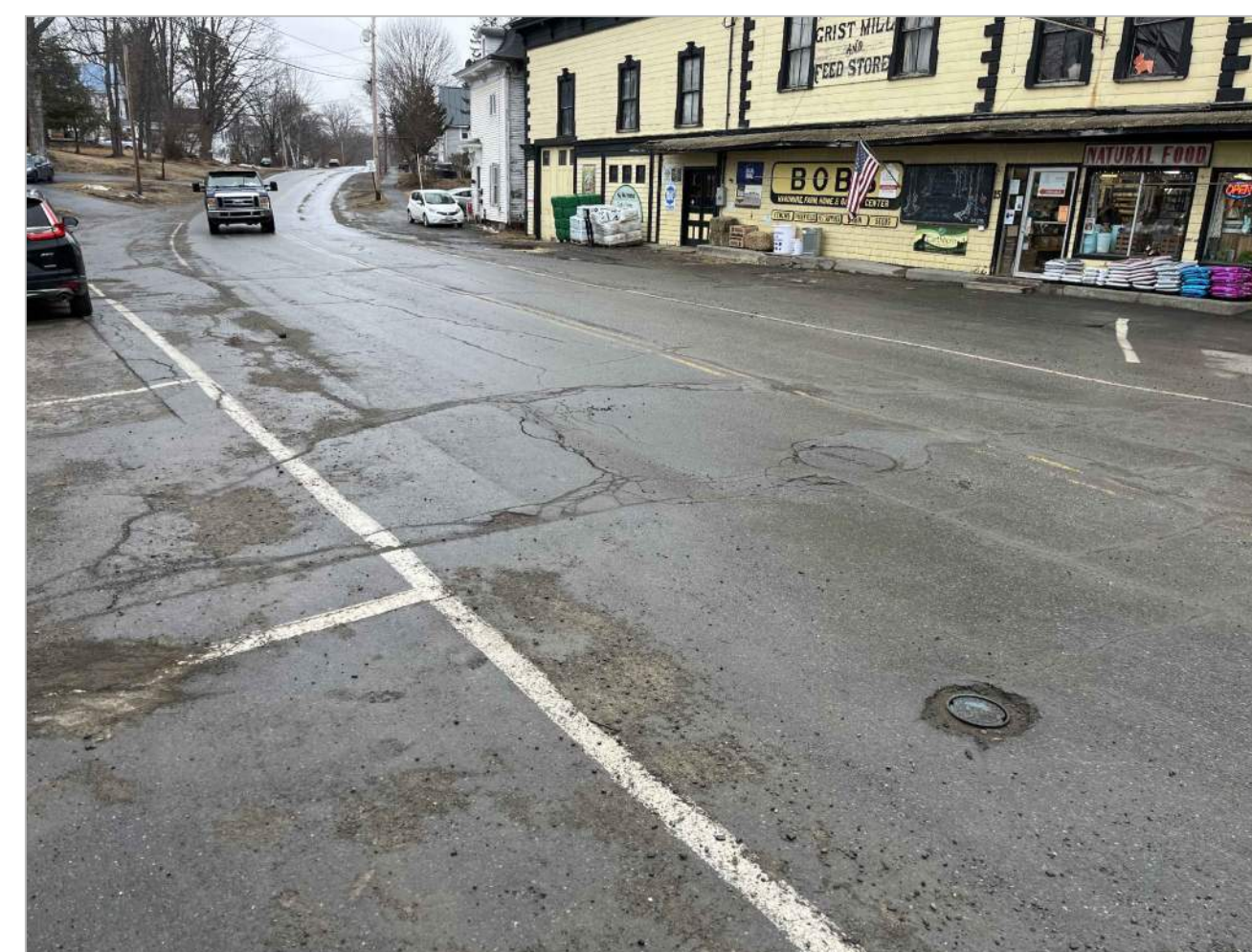
PHOTO 5 LINCOLN STREET WEST APPROACH
