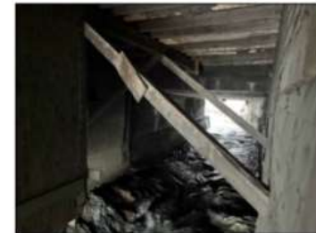
PHOTO 4 DOWNSTREAM LOOKING UPSTREAM
